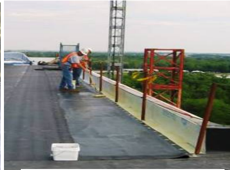
Parapet wall on bridge
