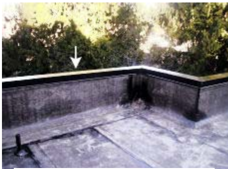
Parapet wall on roof
