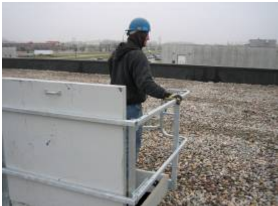
Guardrail, swing gate, and grab bars
